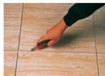
The grouting material should be applied with a rubber trowel. The use of metallic trowels should be avoided at all times, since they may damage the glazed surface of tiles. Grout is available in a wide array of colours, which makes it possible to match the shade of any setting created.
