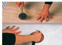
During the installation phase, before setting is complete, it is recommended to continuously check the pieces that are already installed, since there is still time to fix any faults. A rubber mallet can be used to tap down projecting tiles and a suction-cup can be used to pull up pieces that are sunken in excess.
